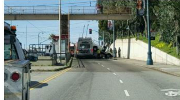
Pedestrian Bridge and retaining wall on Ocean Avenue
