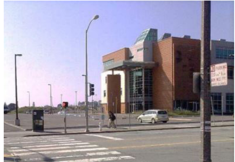
Multi Use Building on Frida Kahlo Way
