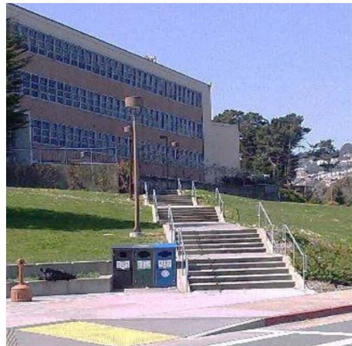
Stair from Cloud Circle to Cloud Hall
